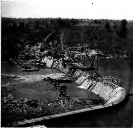
FIG. 4.—POWER DAM ON THE CHATTAHOOCHEE RIVER.
